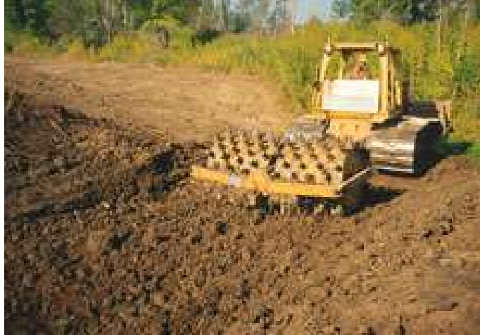
Sheepsfoot Roller to Compact Clay Soils
